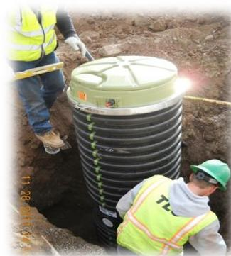
Contractors began working in the neighborhoods by installing the trunk lines within the street areas. Once the trunk lines are installed, the contractor will make arrangements with the property owner for installation of your grinder pump, and to close out the old septic system. The Town realizes that each property is unique and will make sure the contractor does everything possible to respect your wishes and make sure your connection goes as smoothly as possible.
